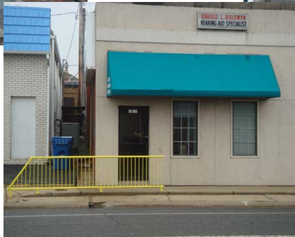
New railing for Audio Hearing Center at 1306 Broadway
