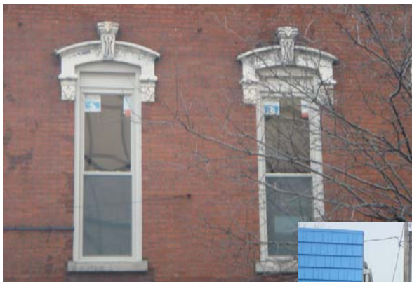
New windows in the J & R Appliance building at 1001 Broadway
